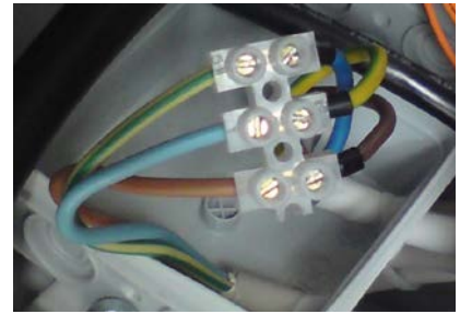
Fig. 7: Here N and PE have been reversed
